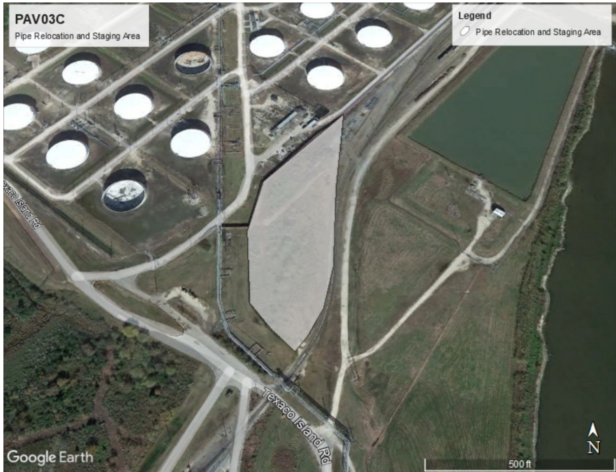
Figure 5. Pipe Relocation and Staging Area for PAV03C
